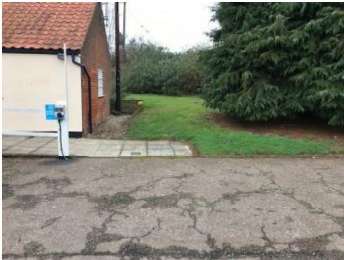
Accommodation Access From Car Park
